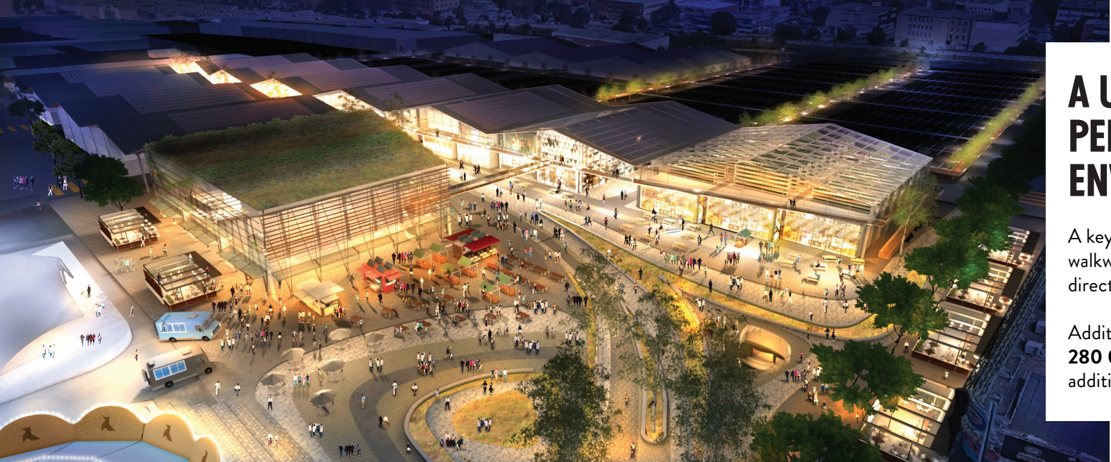
Aerial view of the project
